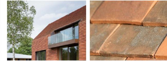
Clay tiles will be utilised on the roof colour matched to selected brick to give a cohesive and clean appearance to the main volume of the building. The choice of clay relates to the potteries history of the area.
