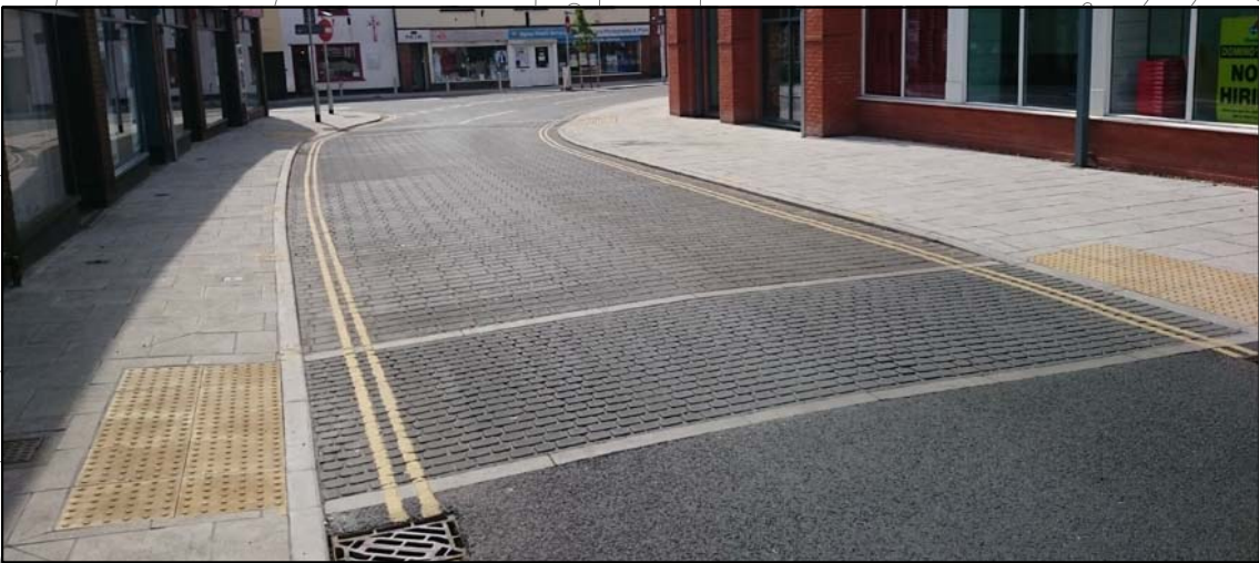
IMAGE 2: IMPRINT SURFACING USED TO REDUCE VEHICLE SPEEDS BY VIBRATION AND CREATE A CONTRASTING SURFACE TO VISUALLY IDENTIFY AN AREA WITH HIGHER PEDESTRIAN TRAFFIC, TIVERTON HIGH STREET
