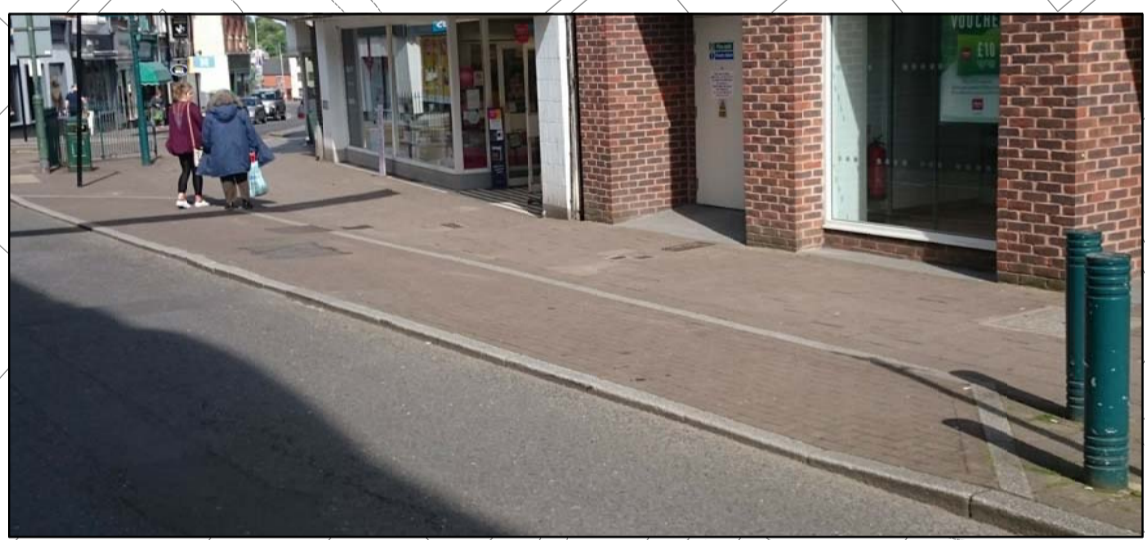
IMAGE 1: ON FOOTWAY LOADING BAY WITH BAY DELINEATED BUT SURFACED SO PEDESTRIANS MAY USE IT WHEN NOT IN USE, TIVERTON HIGH STREET
